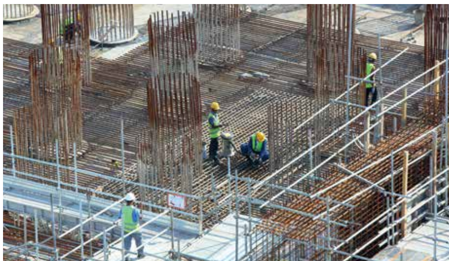
Health and safety practices at "Cinnamon Life" construction site
